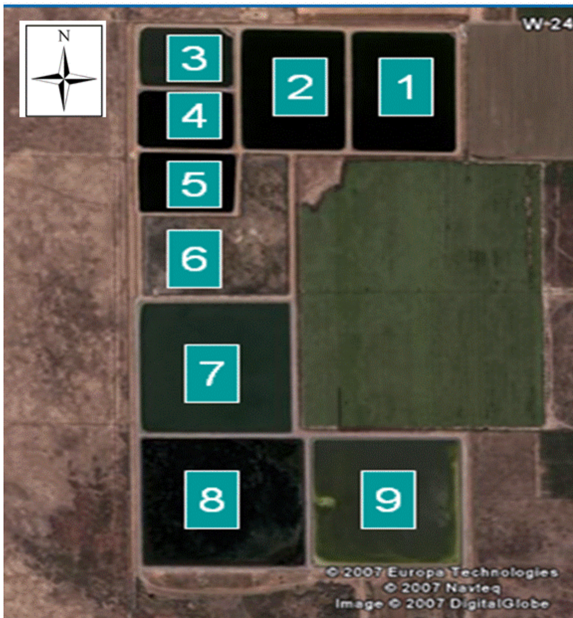
Figure 9 City of Mountain Home Wastewater Treatment Facility Lagoons (adapted from Google Earth 2007)
